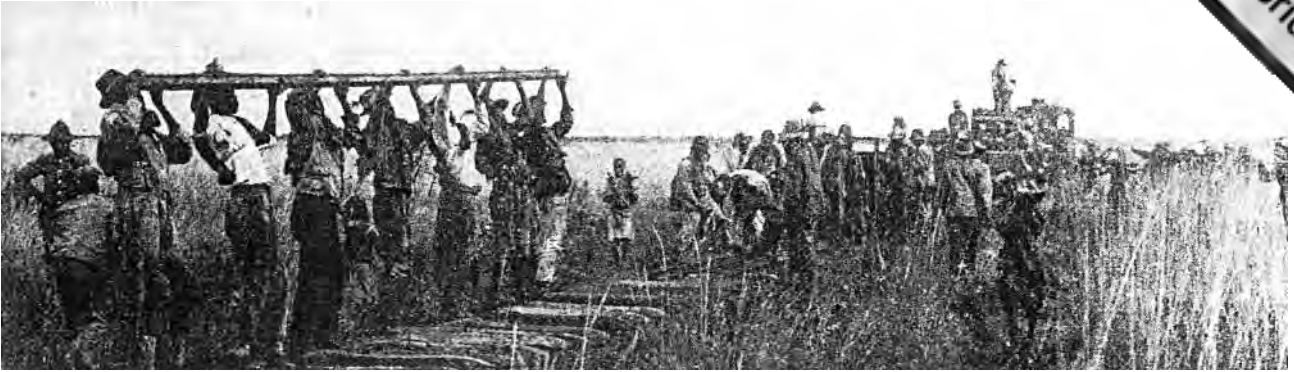
Construction of the Otavi Railway.
